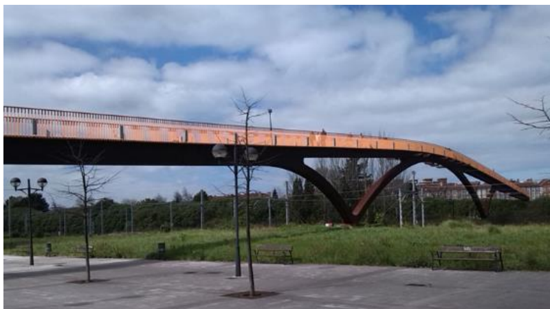
Figure 1. The Pumarín-Moreda footbridge
