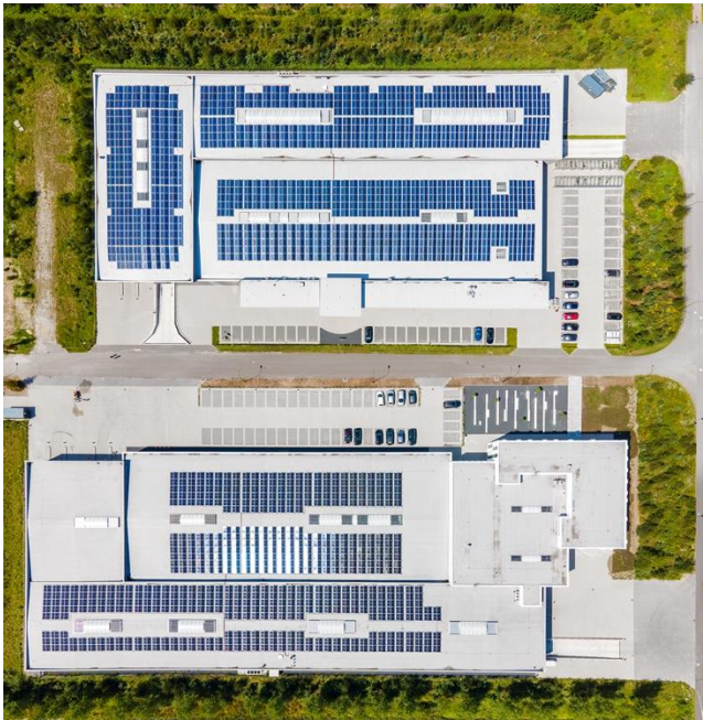
Figure 17, Barco's solar panel installation
