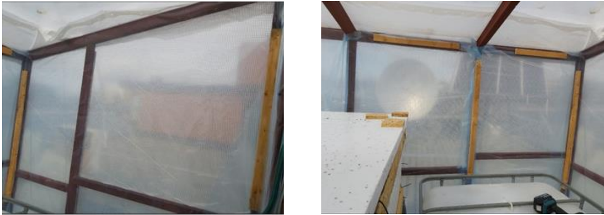
Figure 77. Example of the reinforcements to the inside isolation.
