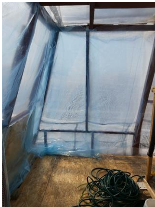
Figure 76. Example of the blue sheets on the inside for insulation.
