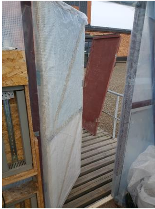
Figure 82. End result of the door.
