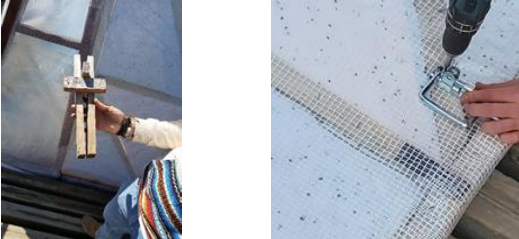
Figure 81. Comparison of the old (left) and new (right) locking system.
