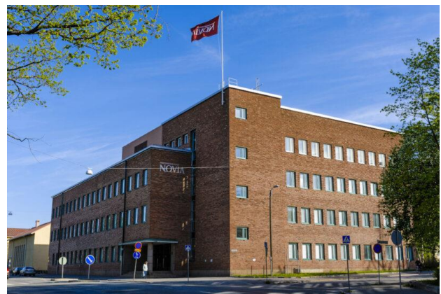
Figure 1.1 -Novia UAS Building
