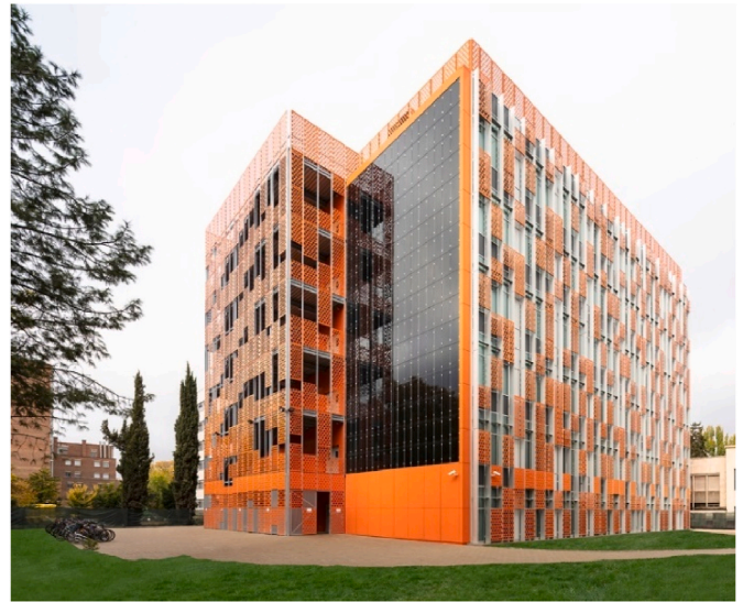
Fig. 3. Profile view “Aulario IndUVa”.
