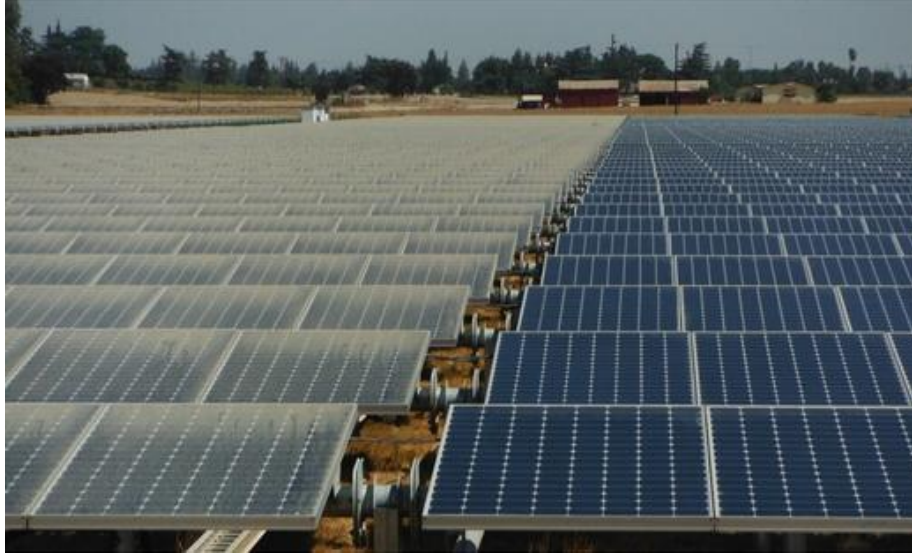
Figure 9. Soiling coming from dust deposition [29].
