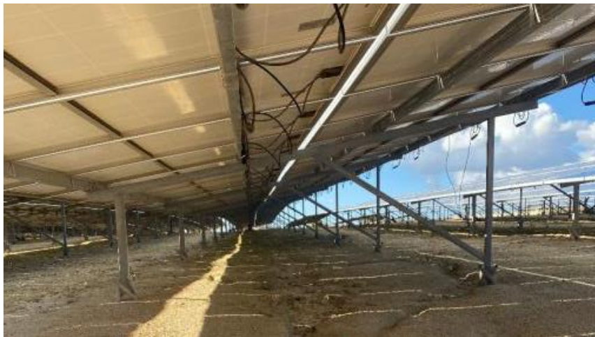
Figure 36. Anchoring of PV modules to the ground in PV Farm 2.
