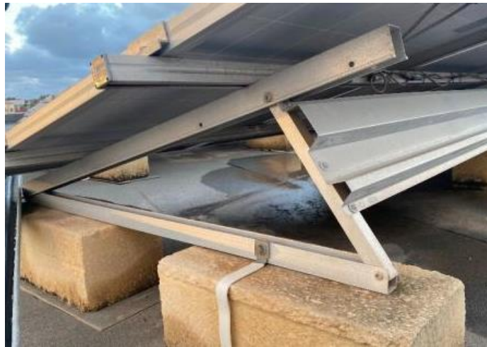
Figure 43. Anchoring A-frames to the roof in first roof of PV Farm 3.
