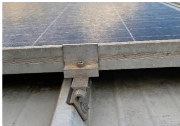
Figure 44. Anchoring with Clampfit in first roof of PV Farm 3.
