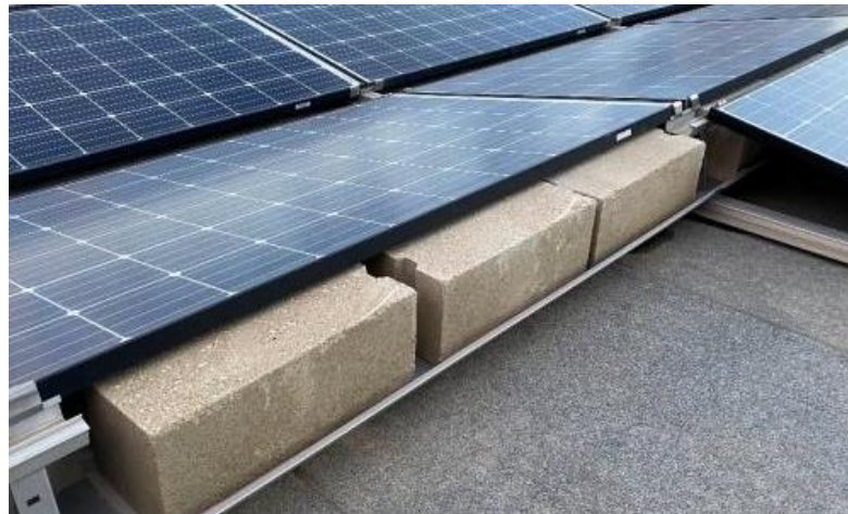
Figure 46. Anchoring with Fixgrid W-E in second roof of PV Farm 3.
