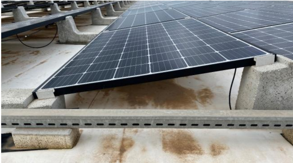
Figure 48. Anchoring to the roof in PV Farm 4.
