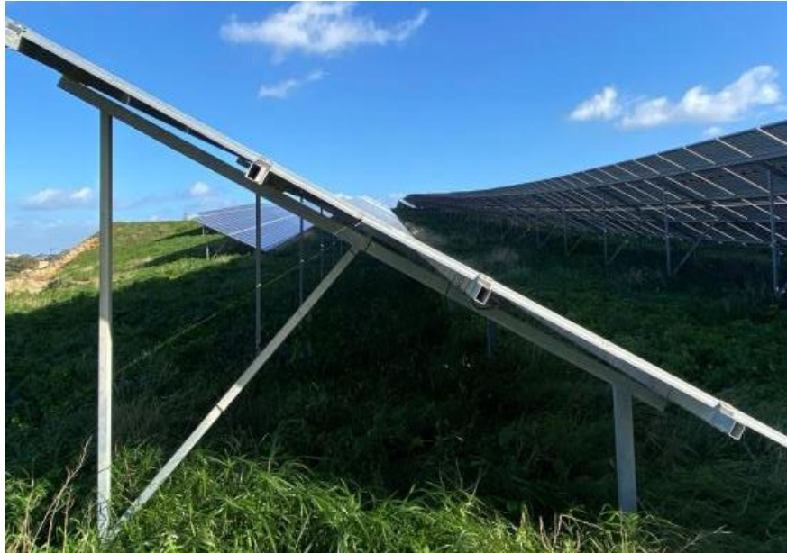
Figure 30. Inclination and orientation of the PV modules at PV Farm 1.
