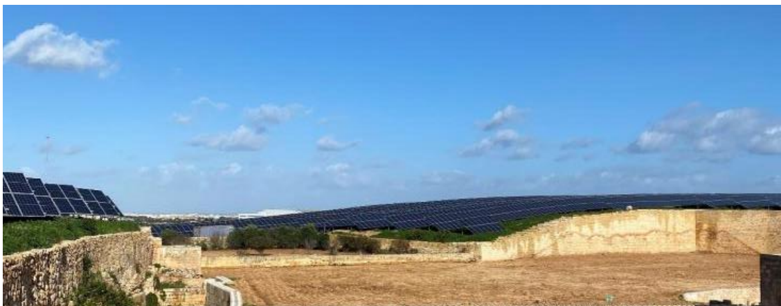
Figure 27. Landscape view of the 1 st PV installation.
