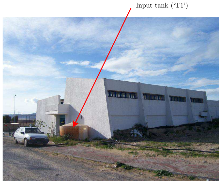
Figure 3.1: Location of the RO pilot plant.
