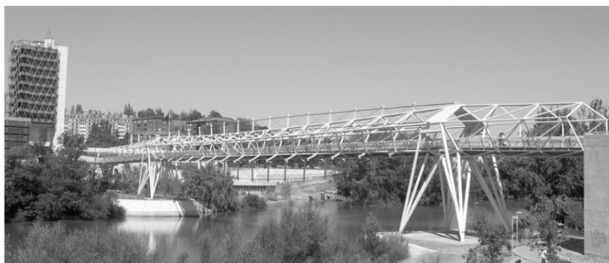
Figure 1: Science Museum Footbridge of Valladolid.
