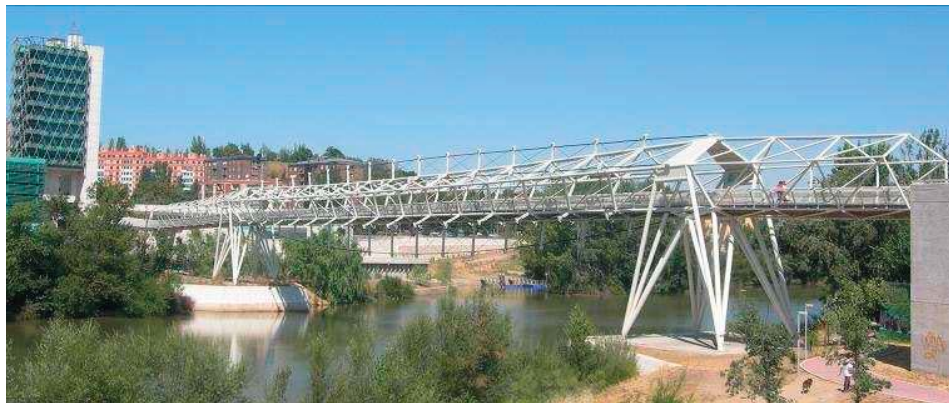
Figure 1. Science Museum Footbridge of Valladolid
