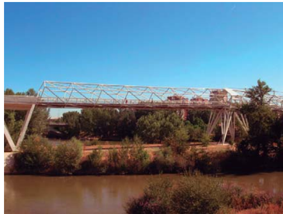
Fig. 4. Science Museum Footbridge.
