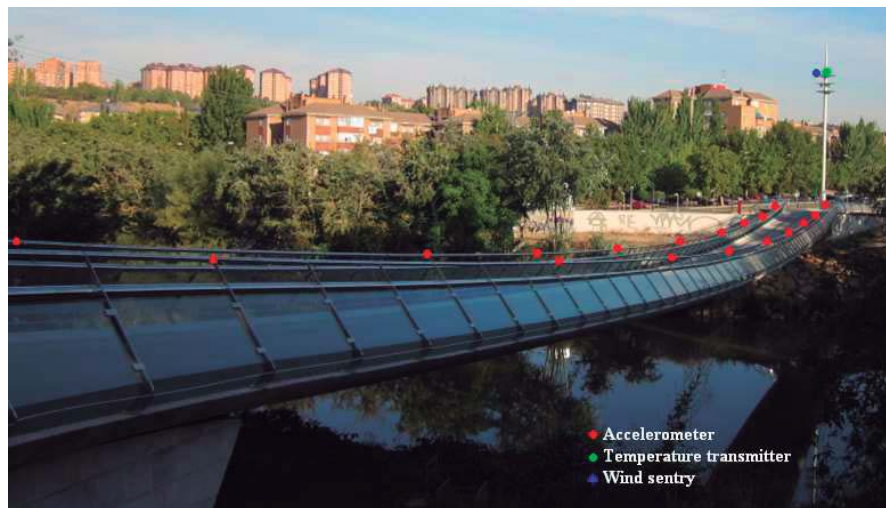
Figure 2: Sensors distribution on the structure.
