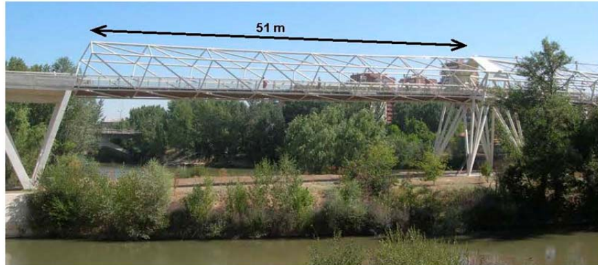
Figure 2. View of Span 2
