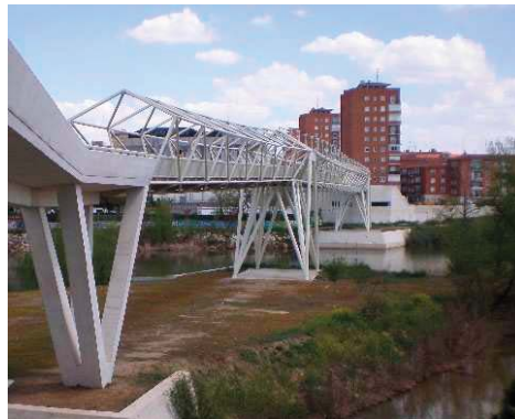
Figure 1: Science museum footbridge of Valladolid
