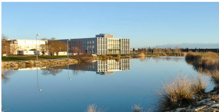
Figure 1. LUCIA near Zero Energy Building (nZEB), Valladolid, Spain.
