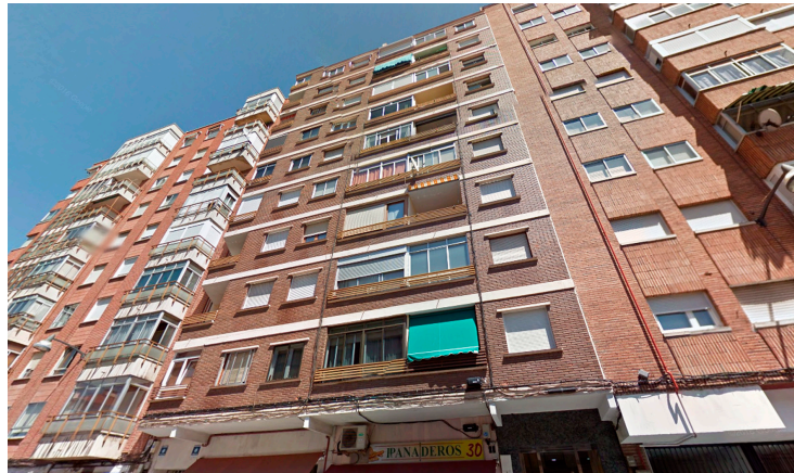
Figure 8. Exterior image of the case study 09683460651630036.
