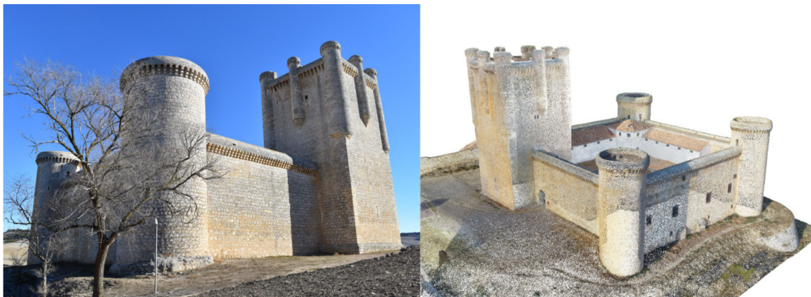
Figure 1. Complete point cloud of the Castle of Torrelobatón into REVIT as RCP.
