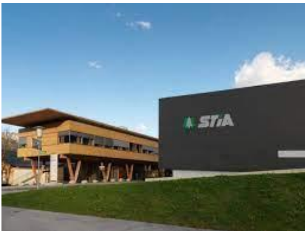
Figure 3. STIA Biomass CHP plant based on an ORC process
