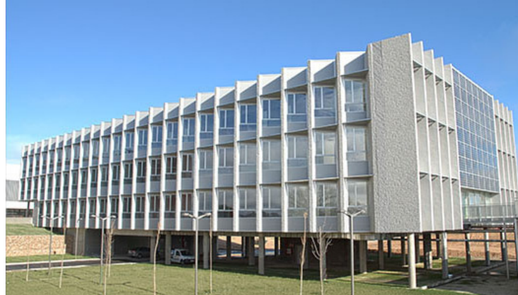
Figure 1. General view of the LUCIA building.
