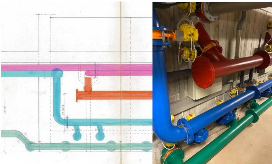
Figure 7.9 (left) and 7.10 (right) shows the filter configuration. The left image is a drawing based on the provided data, featuring a transparent wall that allows for a clear view of the filter. On the right, an actual photograph taken during the visit to Hinnerup Waterworks on May 3rd showcases the real-life appearance of the filter setup.
