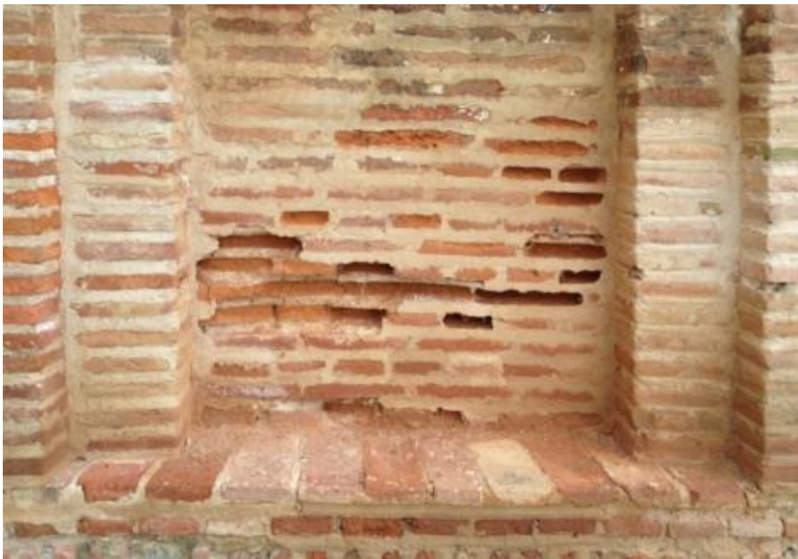
Figure 1. Photograph of a Mudejar-style church facade, where the differences in the states of the brick and mortar joints can be observed
