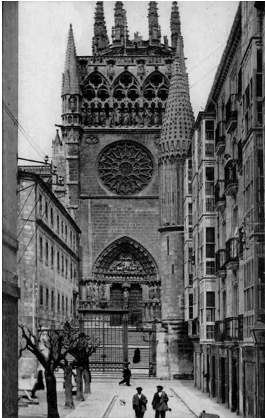
Fig. 9 - General view of the Sarmental's gate after the demolition of the east bay of the palace, where the regularized layout and composition of the new façade and the access railings to the widened staircase can be appreciated. Photograph of the Phototype of Hauser and Menet, Madrid. Source: Digital Library of Castilla y León, symbol: 726.6 (460.182 B).
