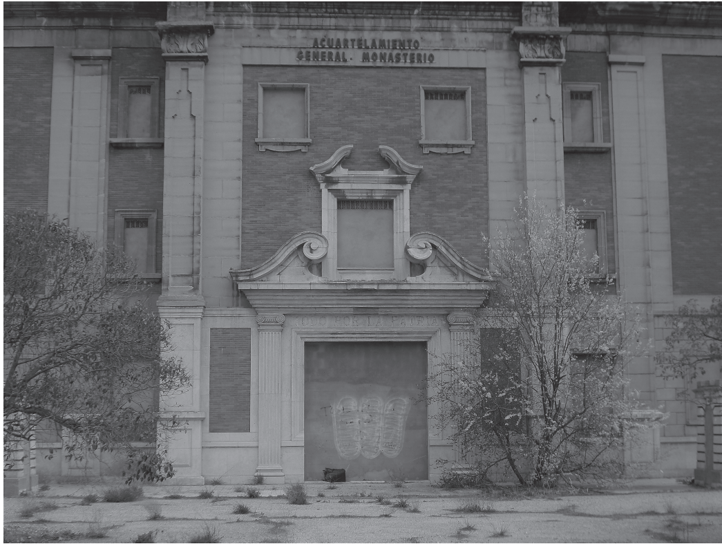
Figure 13.1 The General Monasterio barracks lying abandoned in Valladolid, Spain.
