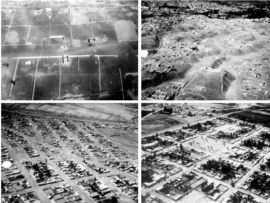
Figure 7: Stages of squatter settlement growth. Source: Turner, 2018: 42, John F.C. Turner Archive, Colegio de Arquitectos de Cataluña.
