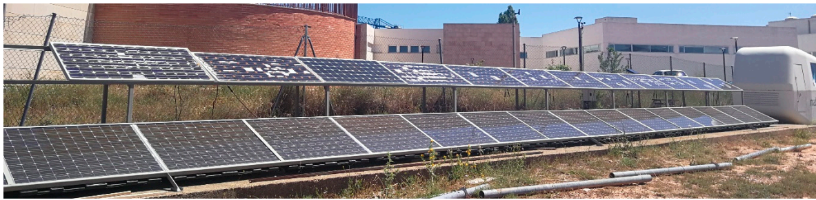
Figure 5. PV field of the Campus Duques de Soria of the University of Valladolid in Soria, Spain.
