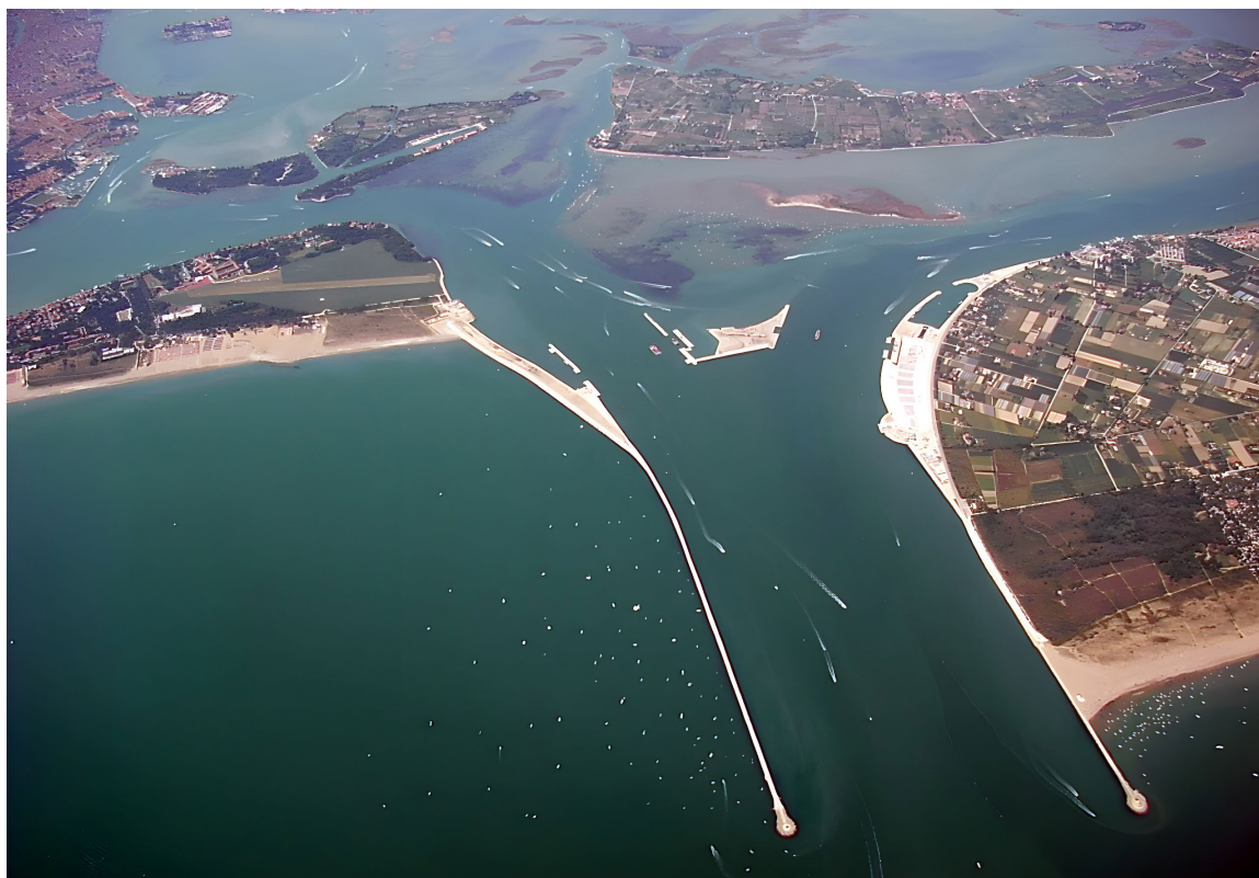
^ Fig. 10 Aerial view of the MoSE project in Venice, Porto di Lido (channel north of Lido) in mid-2009 (Source: Chris 73, 2009. Wikimedia Commons, CC BY 3.0).
