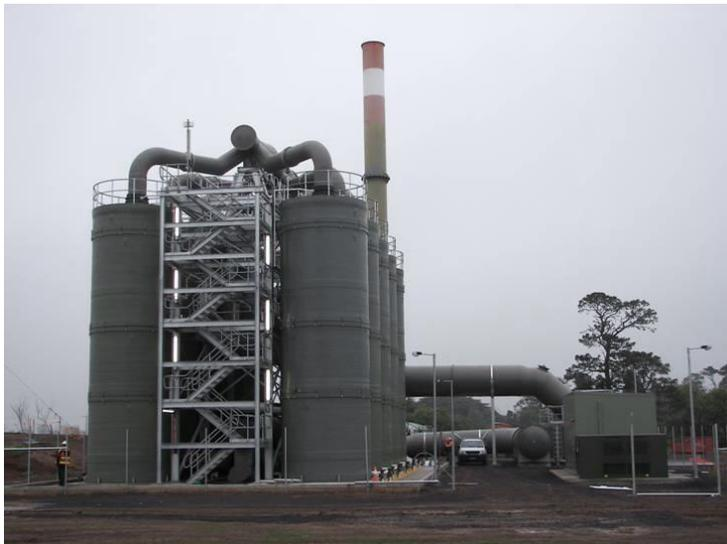
**Figure 3-3** An industrial biotrickling system treating  $126,000 \text{ m}^3 \text{ h}^{-1}$  of foul air from a large sewage interceptor system (courtesy of Melbourne Water, Melbourne, Australia).
