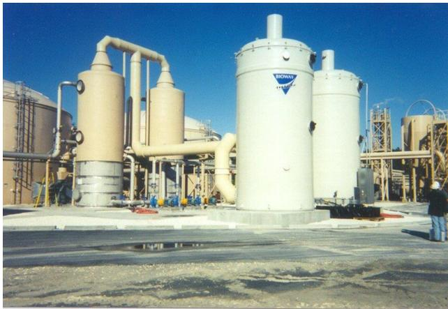
**Figure 3-5** An industrial biological system treating 35,500 m<sup>3</sup> h<sup>-1</sup> of foul air from stripped groundwater at a food processing facility (courtesy of Budweiser, Jacksonville, FL, USA).
