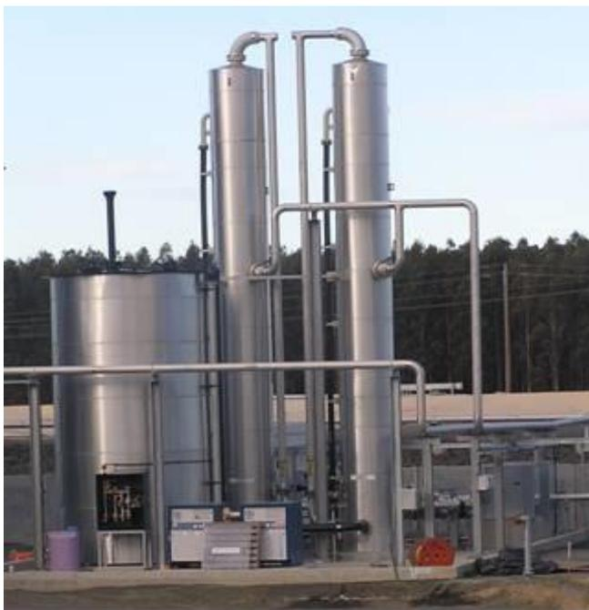
**Figure 3-6** A bioscrubber type system to clean biogas and generate a high value gas for energy generation (courtesy of Gippsland Water, Gippsland, Australia)
