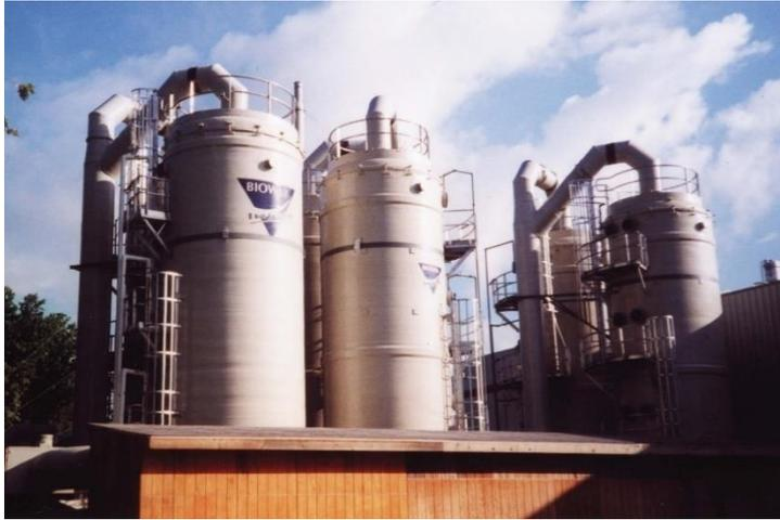
**Figure 3-4** An industrial biological system purifying 51,000 m<sup>3</sup> h<sup>-1</sup> of waste gas from a viscose processing facility and recycling sulfuric acid back to the facility production process (courtesy of 3M, Elyria, OH, USA).
