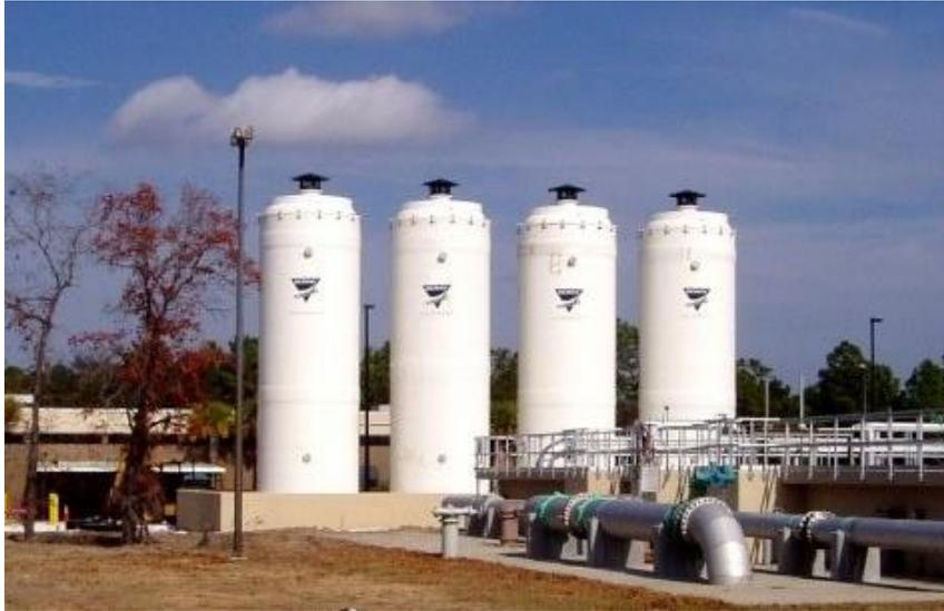
**Figure 3-7** An industrial biotrickling system treating  $47,600 \text{ m}^3 \text{ h}^{-1}$  of waste gas from a water resource recovery facility (courtesy of JEA, Jacksonville, FL, USA).
