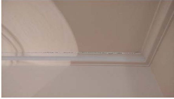
Figure 3.8 Room of the guesthouse under study. False ceiling pathology.
