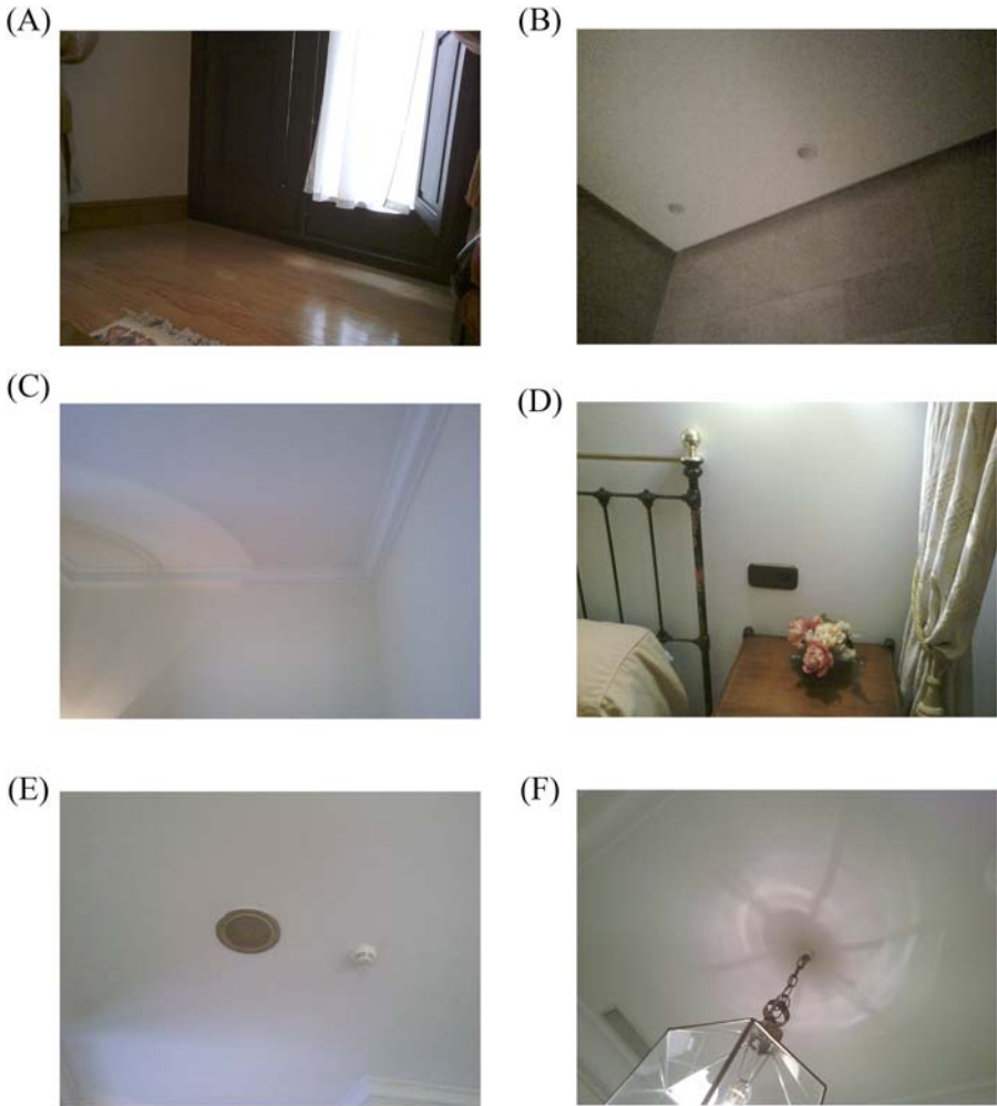
Figure 3.11 Typical leakage paths. (A) Window frames, (B) material joints, (C) wall cracks, (D) electrical grids, (E) ceiling holes for facilities, and (F) plafonds.
