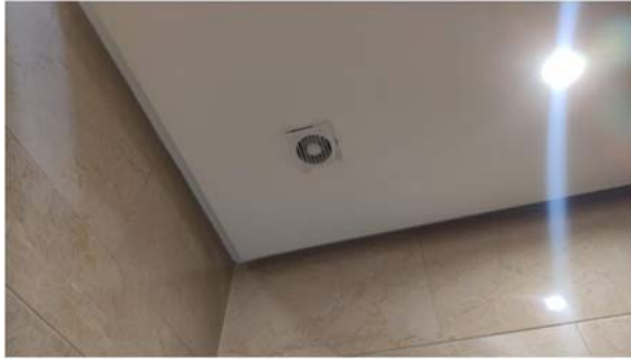
Figure 3.9 Room of the guesthouse under study. Bathroom extraction.
