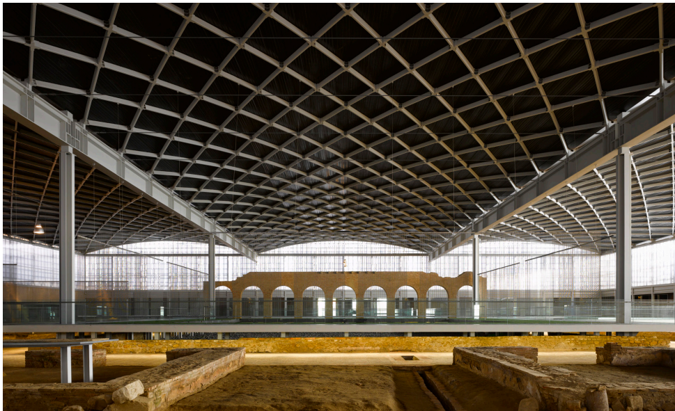
Figura 4.43. Interior nave central Villa Romana
