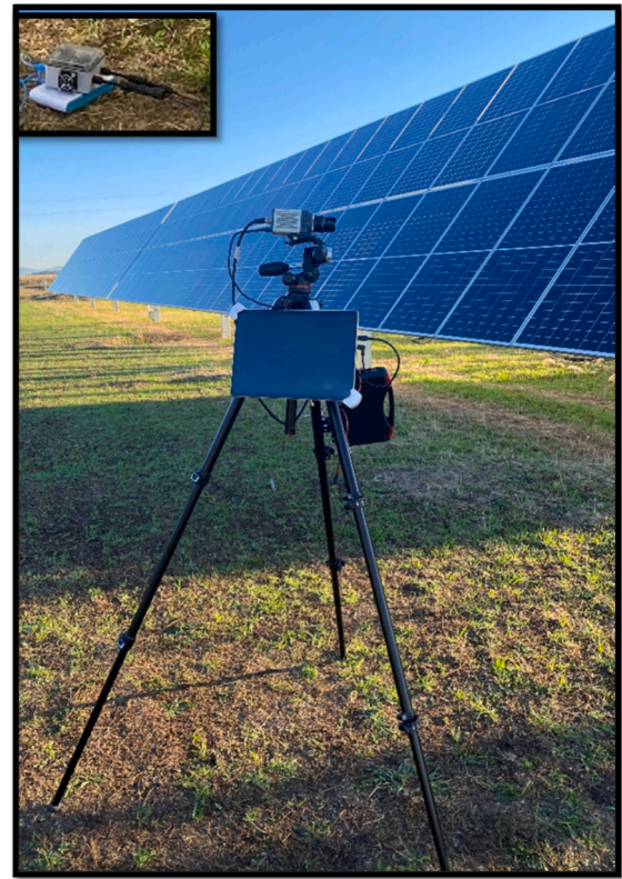
Fig. 2. Set-up used for dEL inspections by the self-powering configuration.
