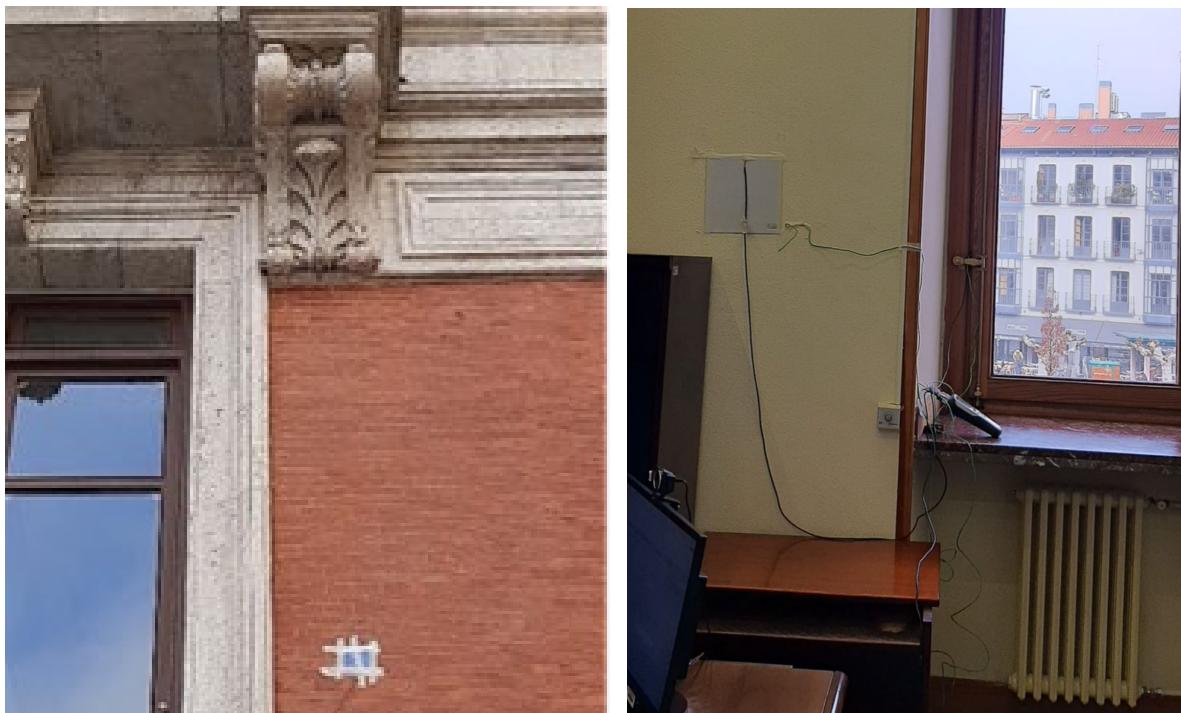
Figure 2. In situ test on the north wall of the Valladolid City Hall, a) Left: exterior plate, b) Right: interior plate (authors' photograph).
