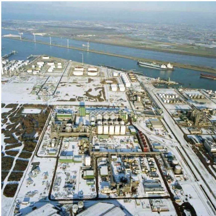
Figure 1: Bioethanol production plant.
