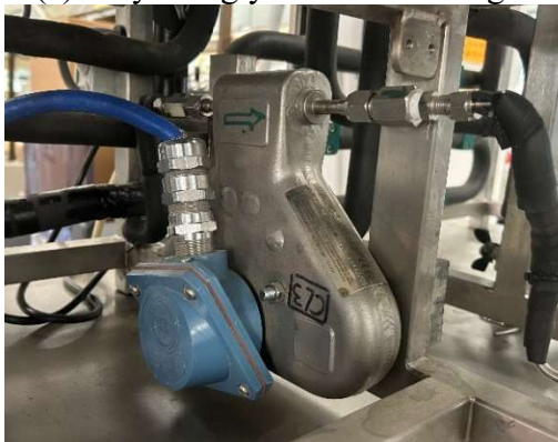
(c) Coriolis mass flow meter
