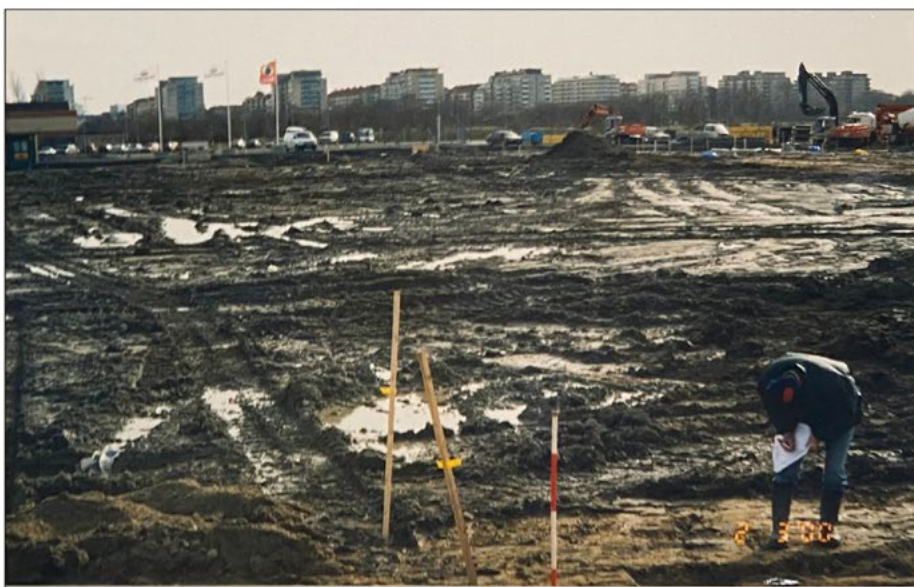
Figure 10: Uncontaminated soil filling the existing polluted land in the southern part of the plot, Sundspromenaden. Malmö Stadsarkiv, box F12:45–50.
