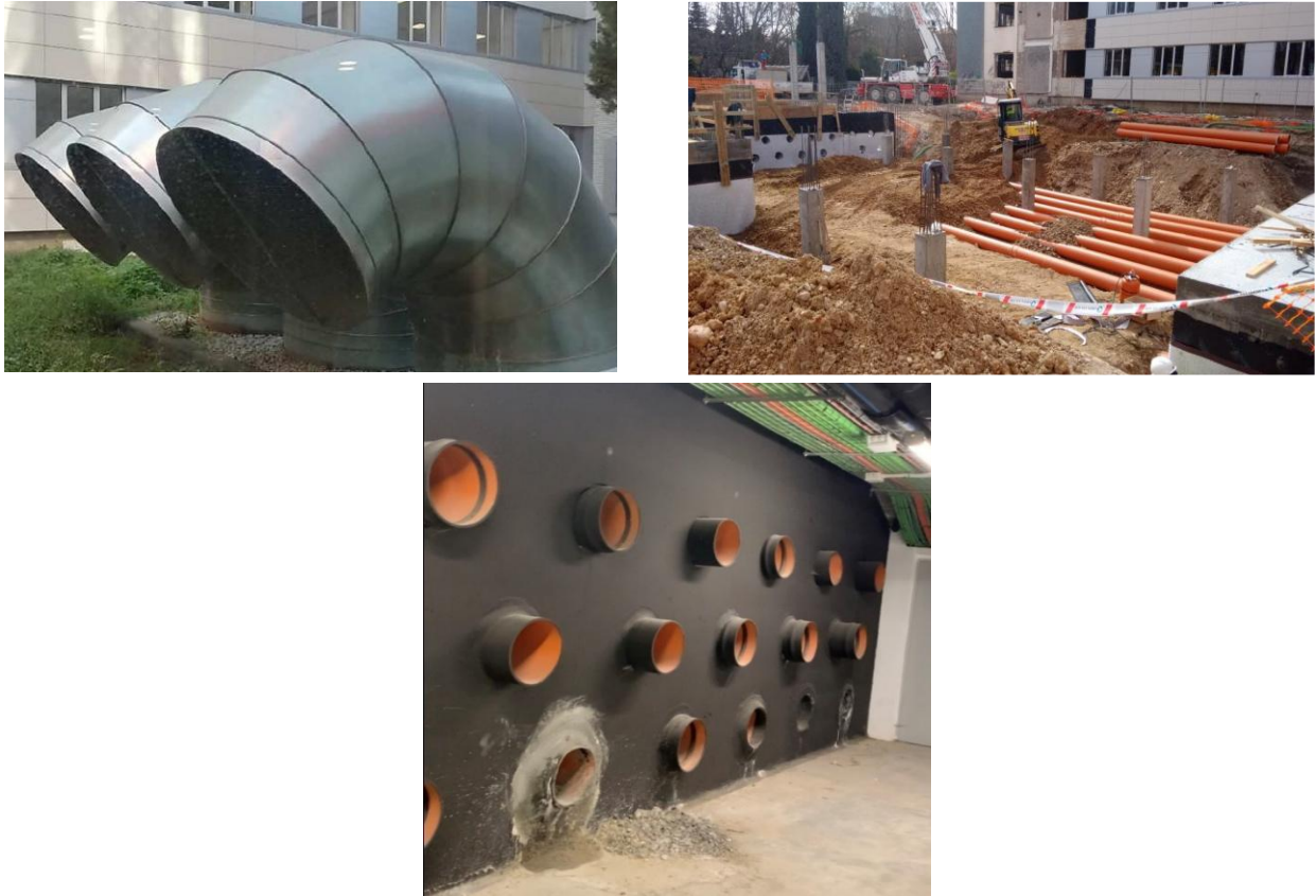
Figure 3.7 Geothermal system (EAHX). View from outside, inside, and installation process
