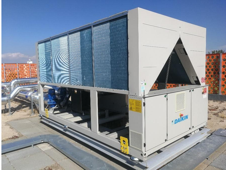
Figure 3.10 Daikin Air-Water Chiller
