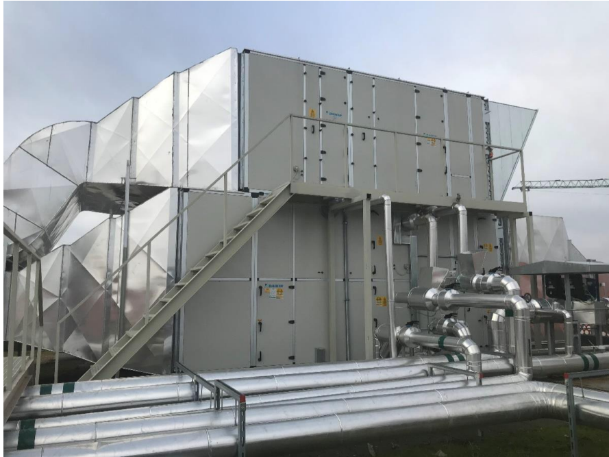
Figure 3.8 Air Handling Unit System (AHU)
