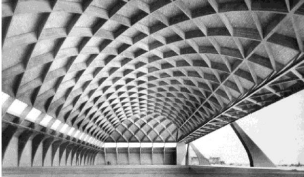
Fig 78. Hangar Orvieto, Pier Luigi Nervi
