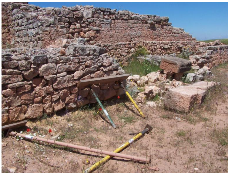
Fig. 1. Archaeological site, previous state. Collapsed walls, uncontrolled growth of vegetation and obsolete fastening elements.
