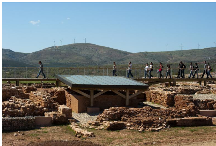
Fig. 3. Joint Forum, reformed state. The consolidation of the north area, with a new protection for the opus signinum tank, made of wood and copper coat. Behind, the wooden bridge.
