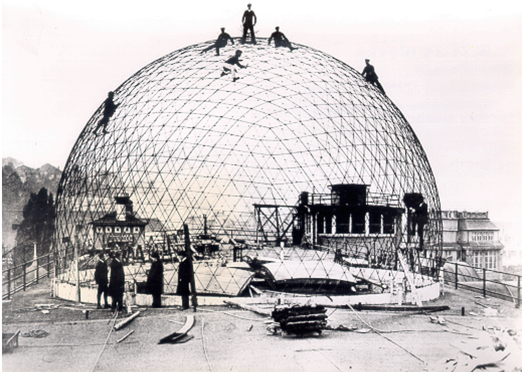
Fig. 1: Construction of a planetarium of Carl Zeiss in Jena (Germany) 1922, planned by Walther Bauersfeld [2].
