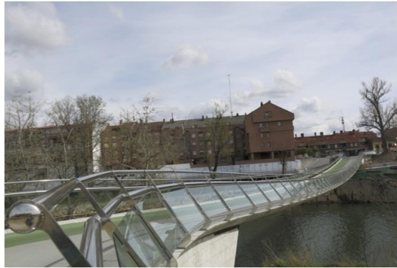
Figure 1. Stress ribbon footbridge under study
