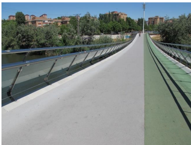
Figura 98. Pasarela peatonal Pedro Gómez Bosque
