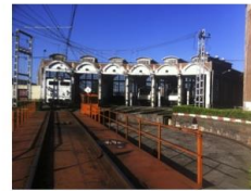
Fig. 3. Cajo-Santander locomotive shed.
