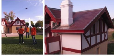
Figure 3: (left) micro-drone flight; (right) image of the roof from its frontal camera.
