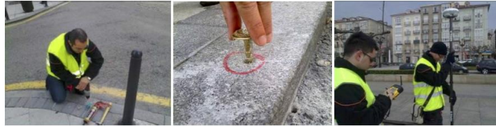
Figure 1. Steps of nail placement on streets for surveying (l-r): drilling, placement and geo-location.
