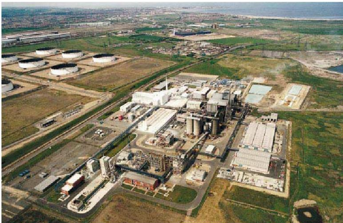
Chloride process factory
