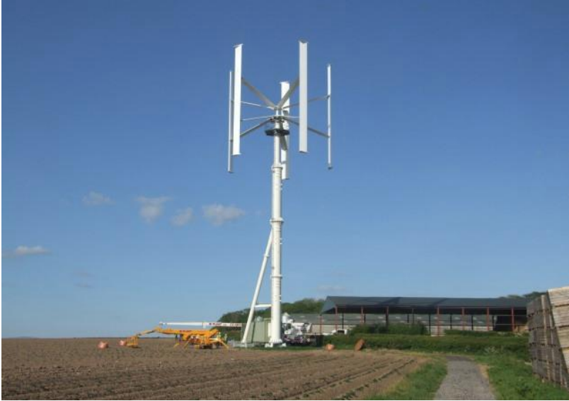
Figure 2.9- Example of a 30-100kW Vertical Axes Wind Turbine in UK ( https://bobbischof.com/about/vertical-axis-wind-turbines-for-micro-generation/ ).
