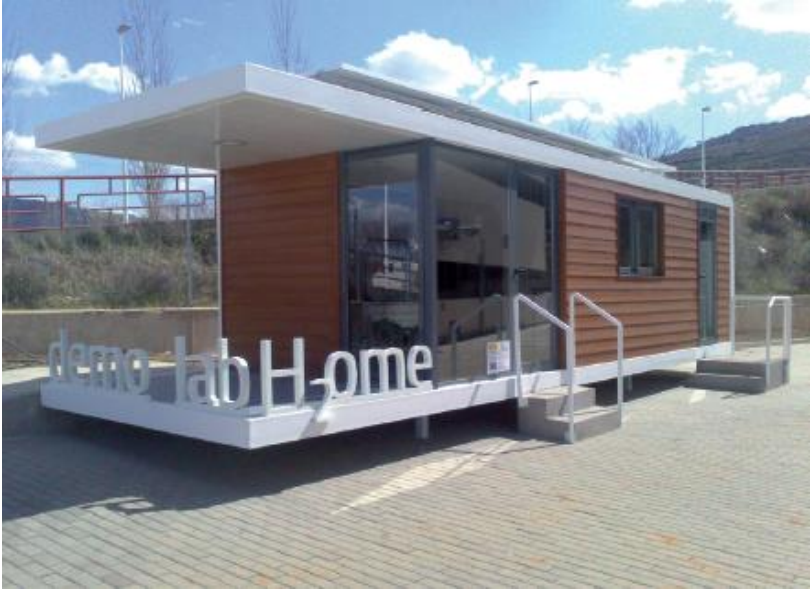
Figure A.2 – Smart house powered by renewable energies and a hydrogen-based microgrid in the CNH2, Spain.
