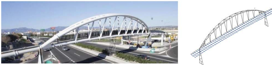
Figure 1. Footbridge under study.
