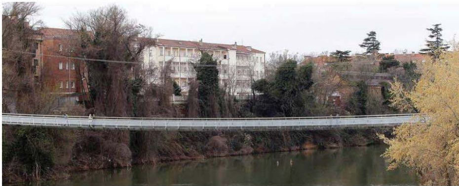
Figure 1. Pedro Gómez Bosque footbridge. Landscape view.
