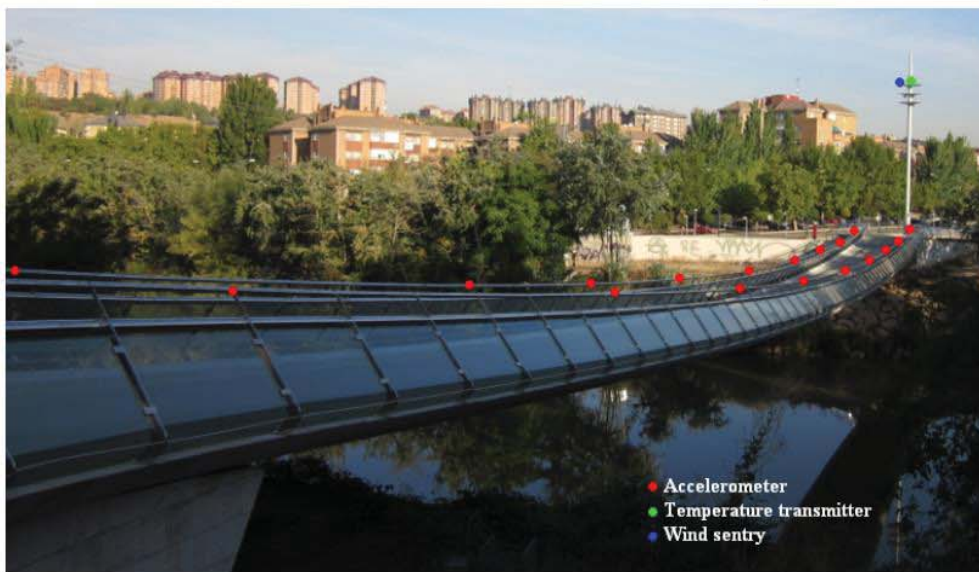
Figure 2. Sensors distribution on the structure.
