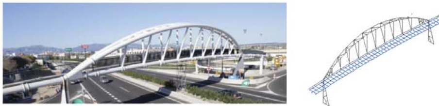
Fig. 1: Footbridge under study: photograph and numerical FE model
