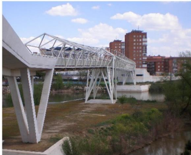
Figure 1: Science museum footbridge of Valladolid
