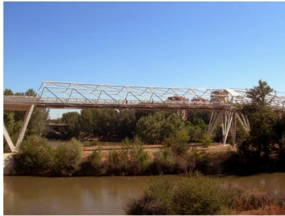
Fig. 4. Science Museum Footbridge.
