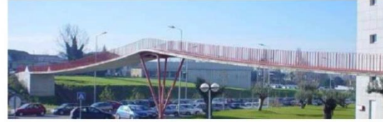
Figure 3. General view of the Stress-Ribbon Footbridge (obtained from [11]).
