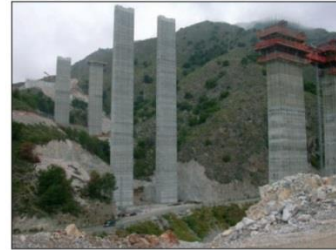
Fig. 1: “La Miel” Viaduct. Malaga, Spain
