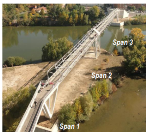
Fig. 1 General view of the test structure
