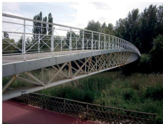
Figure 1. "Isla dos aguas" Footbridge in Palencia (Spain).
