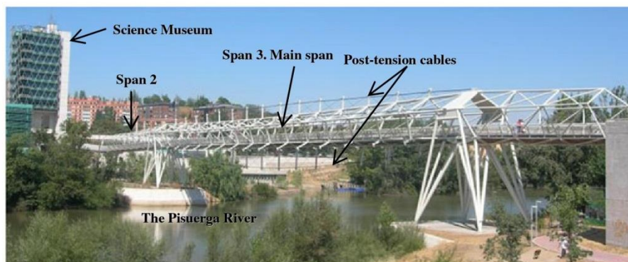
Figure 1. General view of the test structure.
