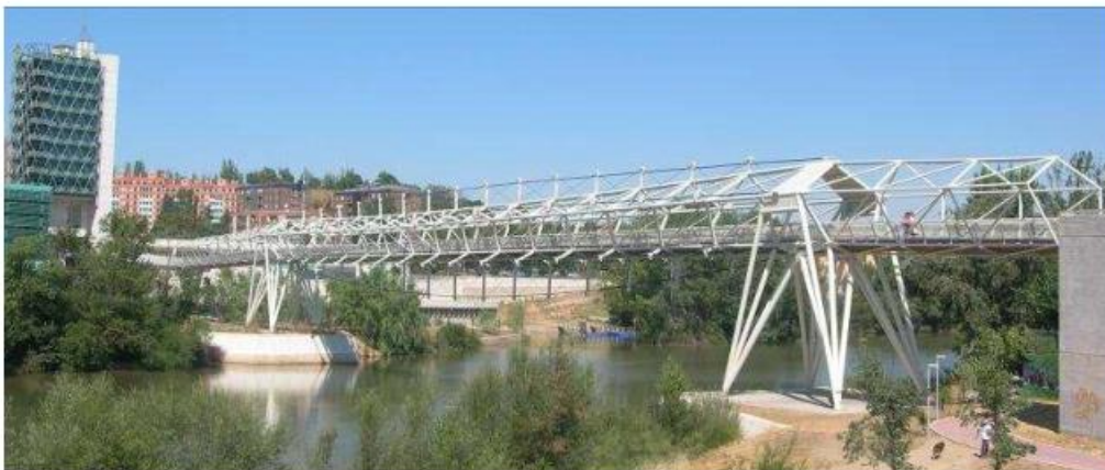
Figure 1. Science Museum Footbridge of Valladolid
