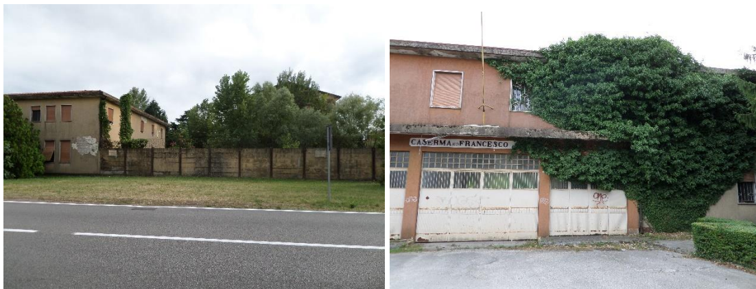
Fig. 64 and 65: the Zanusso barracks before the partial reuse as refugee reception centre.
