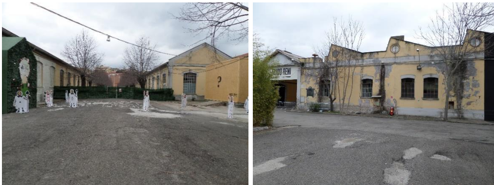
Fig. 45 and 46: two photographs of the former Precision Electrical Components Factory. On the left, temporary activities carried out in 2017. On the right, state of degradation of some buildings.
