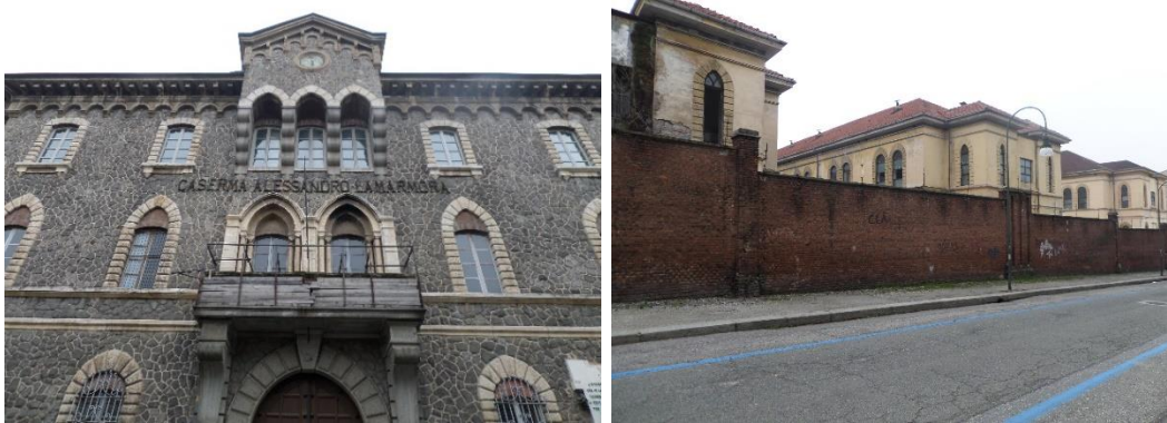
Fig. 56 and 57: images of the exterior part of the La Marmora barracks.
