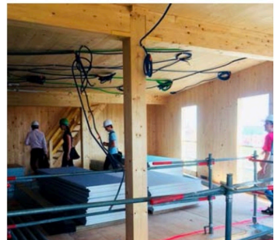
Inside view of the structure Portail de BOIS LAMELLÉ https://n9.cl/hf2r
