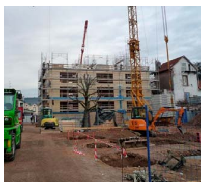
Assembly of the rest of the structure ASP architecture
