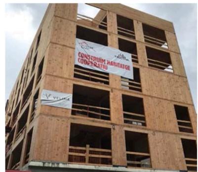
Completed structural phase. Miguel Ángel Rodríguez Nevado
