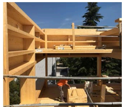
Glulam elements in the façade and CLT floors Miguel Ángel Rodríguez Nevado
