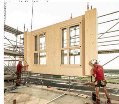
Construction process. Prefabricated façade panel. cetus.at + Thomas Lerch https://n9.cl/4aei7
