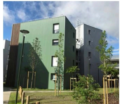
Back façade. https://n9.cl/jehzo
