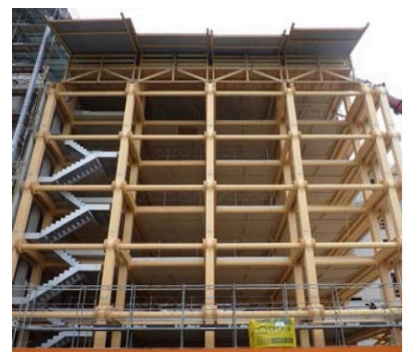
Construction process. Post and beam structure Shigeru Ban Architects https://n9.cl/buizf
