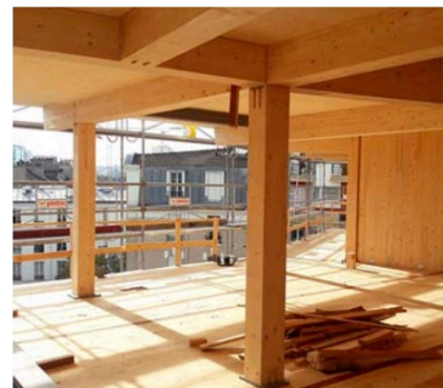
Construction process Sequences Bois https://n9.cl/ivq7x
