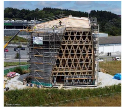
Aerial view. Impulso Verde under construction.
