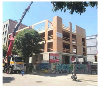
Structure assembly. Miguel Ángel Rodríguez Nevado
