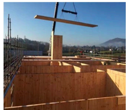
Construction process. Carmelo Fernández Militino
