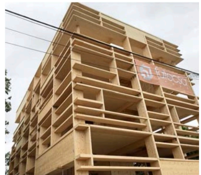
Construction process from the exterior Miguel Ángel Rodríguez Nevado
