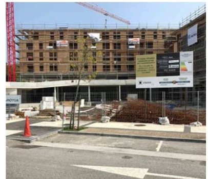
Construction process. Luis-Alfonso Basterra Otero
