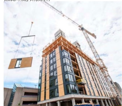
Construction process, façade assembly. Naturally:wood wood https://n9.cl/th0mp
