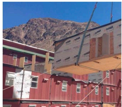
Assembly of prefabricated timber modules ASAP https://n9.cl/bh75d
