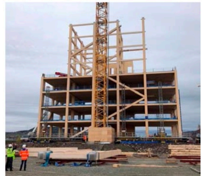
Construction process. First CLT floors and GLT posts. Mjøstårnet https://n9.cl/nux9
