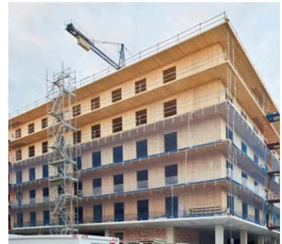
Construction process from the exterior. Egoin https://n9.cl/g4p21
