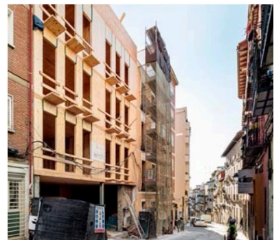
Buenavista Street during construction. B720 https://n9.cl/m2blt
