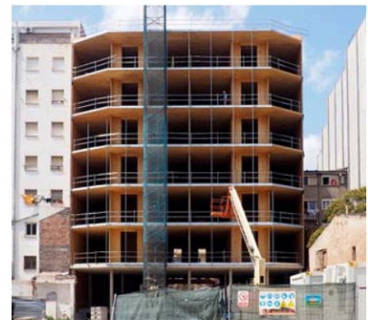
Construction process from the outside. LACOL
