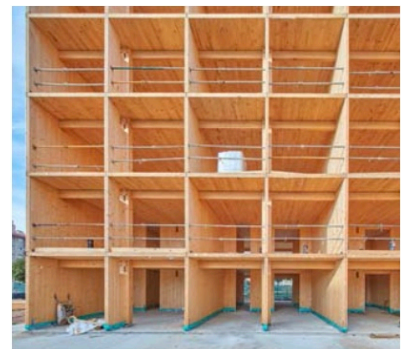
Structure construction process. CLT panels. Afasia https://n9.cl/tx49
