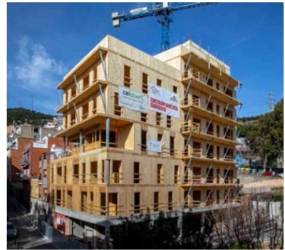
Construction process seen from the outside. Celobert https://n9.cl/usi5
