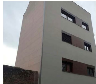
Main façade. House Habitat https://n9.cl/l673i
