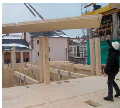
Assembly of the second floor ASP architecture
