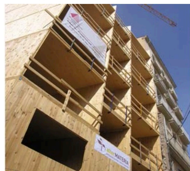
Construction process. CLT panels. Trass Arquitectura
