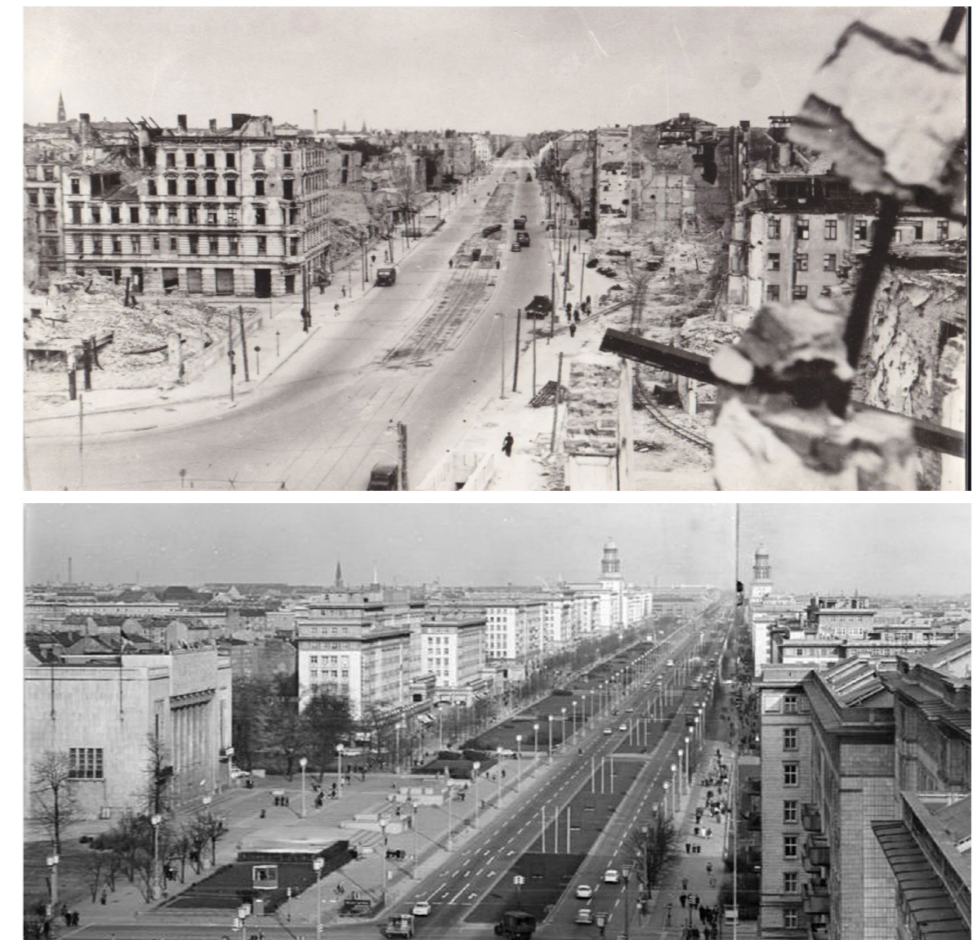
Fig. 44. Top: Große Frankfurter Straße in 1945 with its tram infrastructure. Source: https://fhzz.de/der-rabenstein-strausberger-platz/Friedrichshainer-Zeit-Zeiger . Bottom: Stalin Allee (later Karl-Marx-Allee), reconstructed according to 1952 town planning principles. Source: Federal German Archives (1967a) Bild 183-F0413-0013-001, photo by Koard Peter, 13 April 1967.
