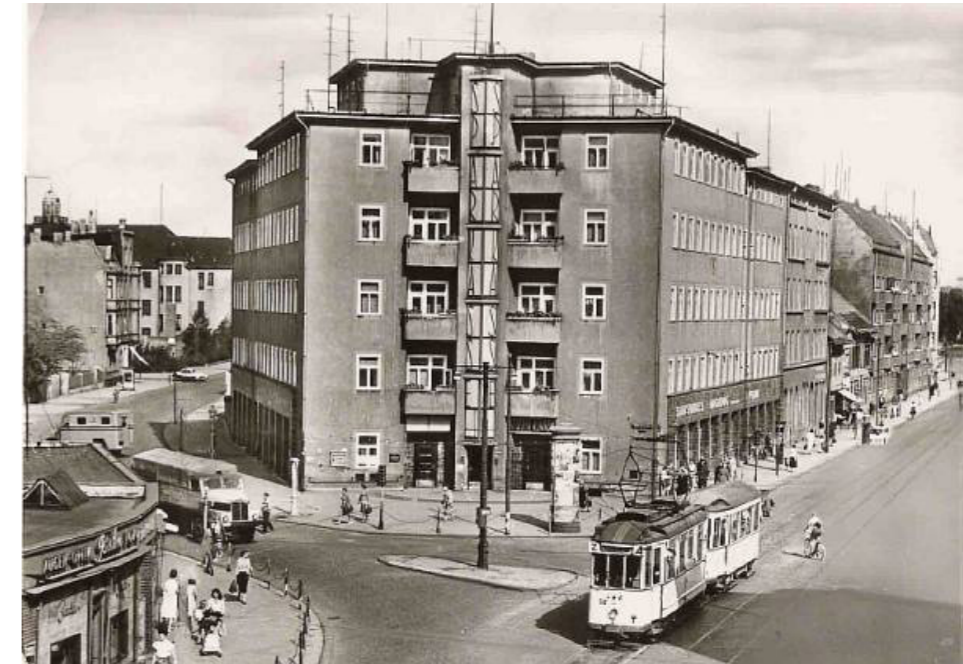
Fig. 10. The new residential area Große Diesdorf in Magdeburg with tram line access in the 1920s. Source: https://www.ddr-postkarten-museum.de/ .
