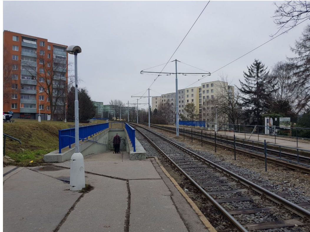
Fig. 226. Pedestrian crossing at the Dunajská tram stop, residential area of Bohunice, organised at a later stage due to the inconvenience of the pedestrian tunnel. Source: Author's photo, 2020. A small change in level can also be seen between the tram stop and the residential area.
