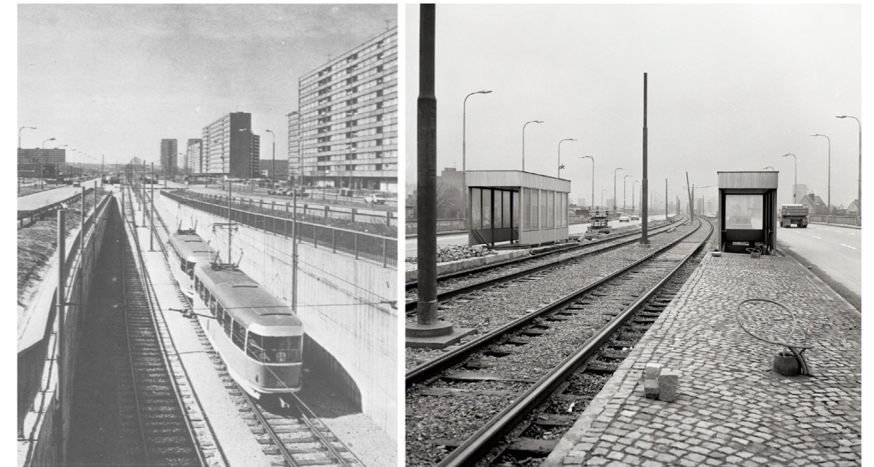
Fig. 156. Images of the rapid tramway in Ostrava in the late 1970s. Left: one of the few underground tramway solutions implemented in Ostrava, in the Třída Dr. Martinka Ostrava-Hrabůvka area in the late 1970s. This type of solution was mainly a solution in intersections with regional roads. Right: reconstruction in 1978 of the Dolní stop in the consolidated city ( Plzeňská Street ). The implementation of pedestrian tunnels to cross tramline in roads with heavy traffic. Segregated tram platforms located in central part of roads was the most widely applied solution in Czechoslovakia during the 1960s and 1970s. Sources: Utvař dopravního inženýrství města Ostravy (1982) Doprava a Životní Prostředí v Ostravě , Ostrava: UDIMO, 10; www.transphoto.com
