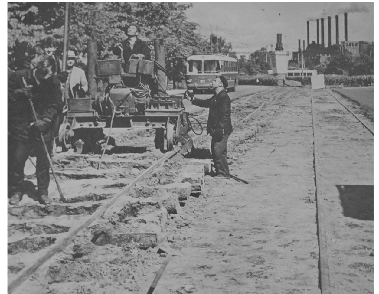
Fig. 158. Sovetskaia Street in the city centre in 1966: removal of tramway line. Source: YarGET Museum.
