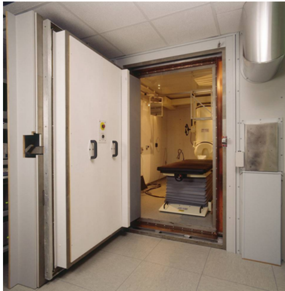
Figure 2.8: Example of magnetically shielded room.
